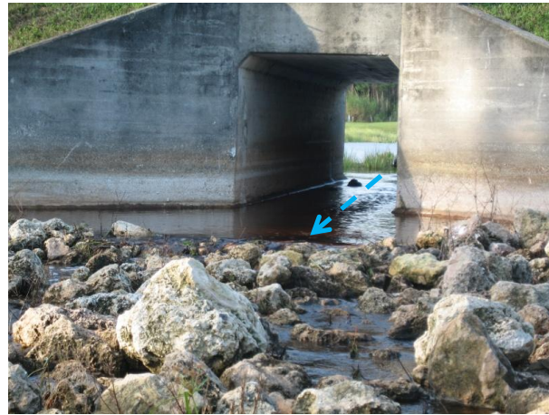
b. Pond 1 discharge through box culvert
