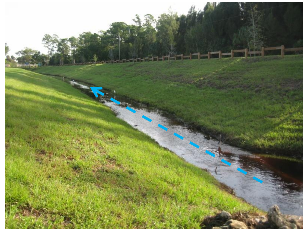
d. Discharge channel under high flow conditions
