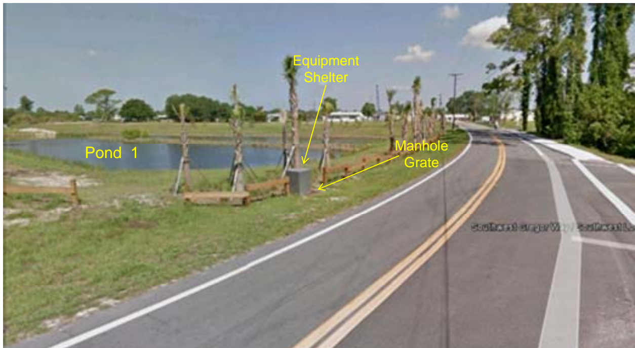
Figure 3-7. Photograph of the Site 2 Monitoring Equipment.
