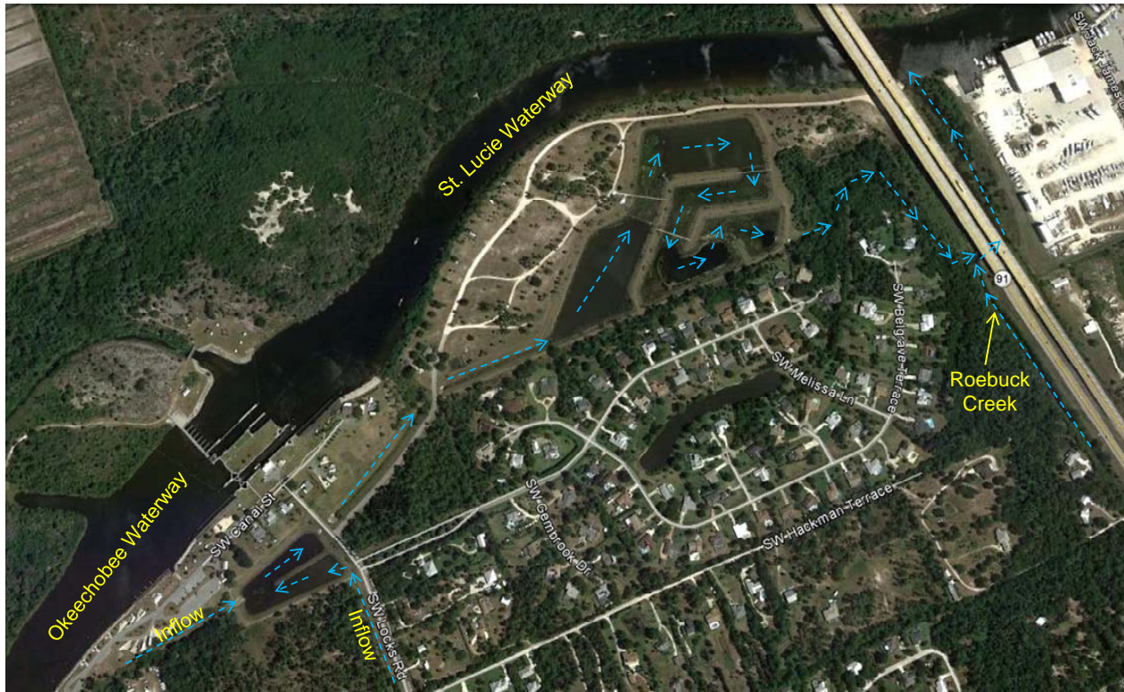
Figure 1-3. Overview of the Tropical Farms Retrofit Project.
