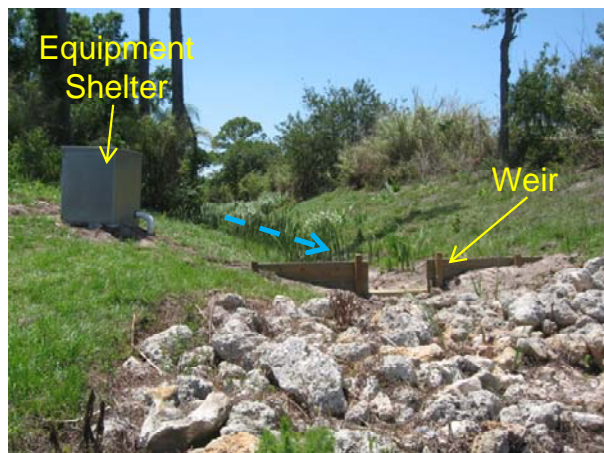
a. Inflow channel with weir structure
