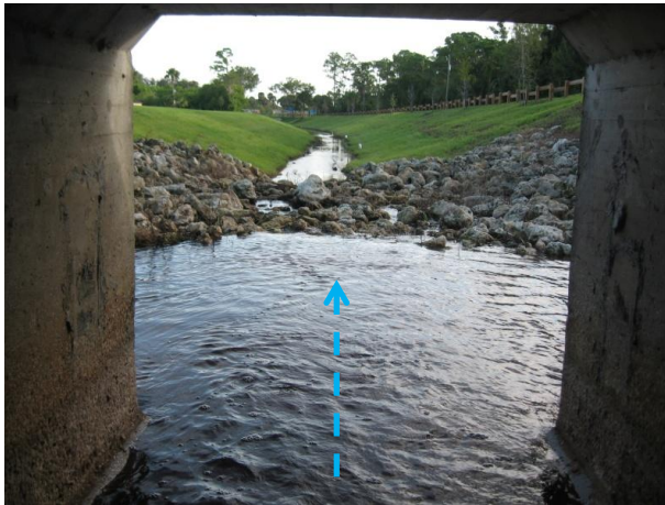
c. Box culvert discharge into channel
