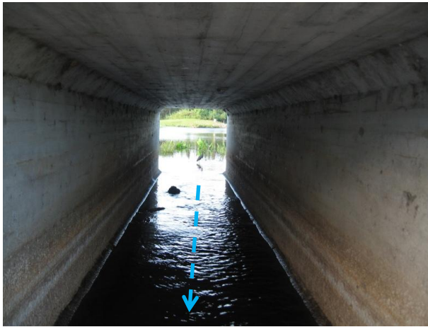
a. High level discharge from Pond 1 through box culvert
