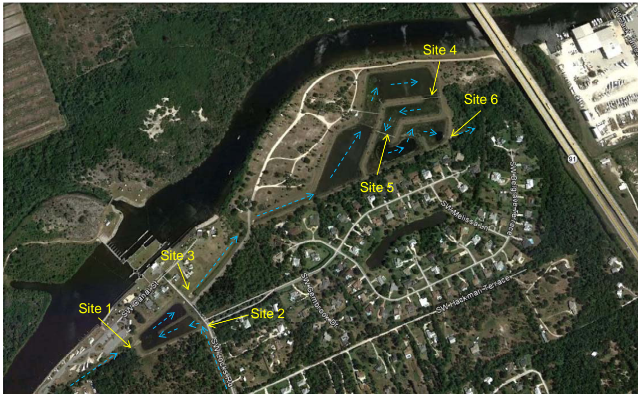
Figure 3-1. Overview of Inflow and Outflow Monitoring Sites at the Tropical Farms Site.
