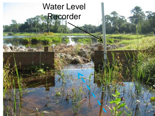
d. Water level recorder
